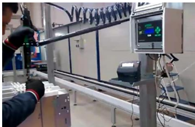
Process under control and print of tightening results
